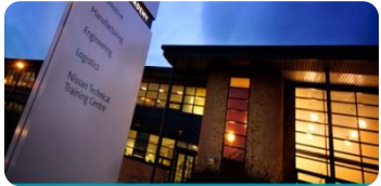
SASMI building (UK)
