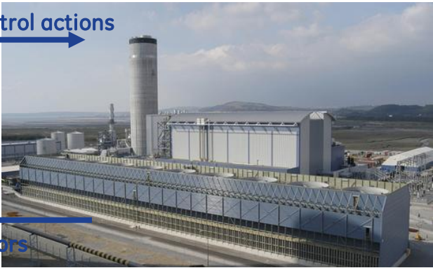
500 MW power plant
